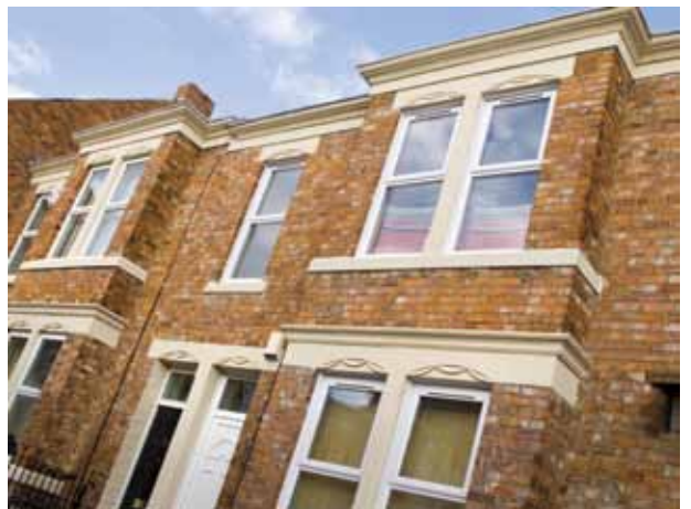
The 'hung windows' on Windsor Avenue are in keeping with the area's traditional style
