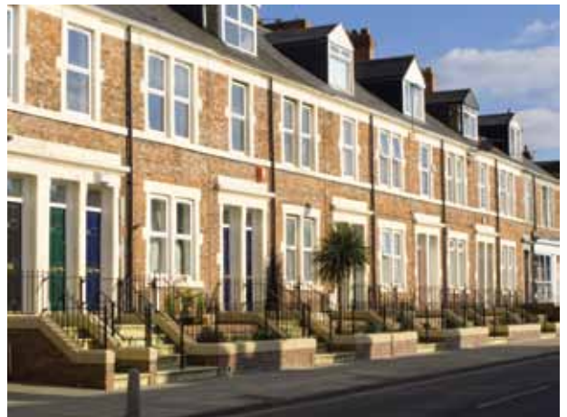
Black rainwater pipes finish off the improvements on Saltwell Road
